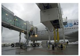
Chillers provide advanced thermal management solutions in various processes. Above are two Jetway air handling units used to provide cool air flow during pre-flight and loading of the aircraft which dramatically reduces fuel and operating cost.
