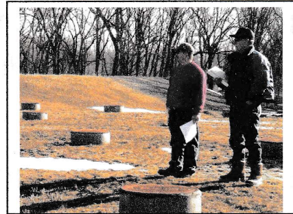
Kelvin Penrod (l) explains the tanks of the Treatment Plant to Marvin O'Grady
