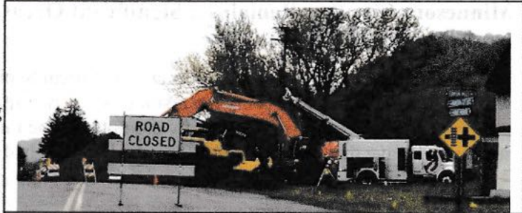
Construction on Bridge Street (Old Highway 61) on April 25, 2012
