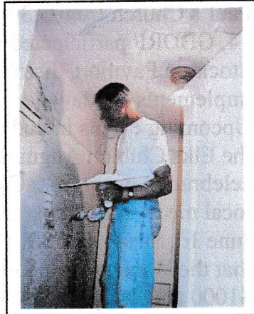
Jim Schoen plasters at the Historic First Baptist Church.
