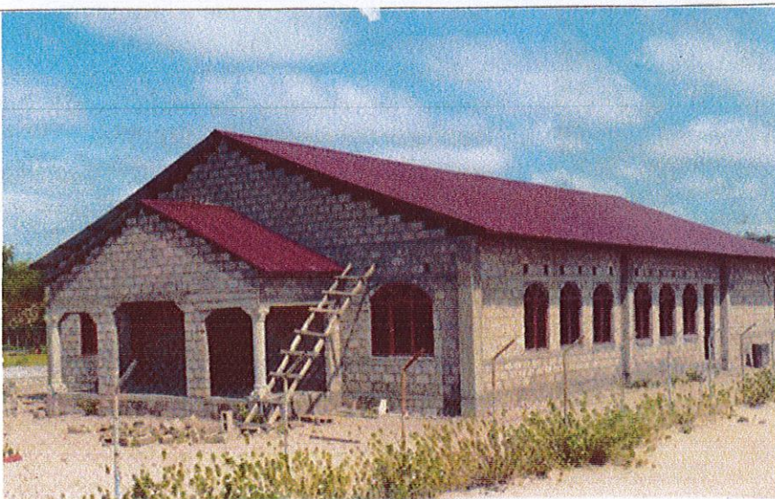
Their building is almost finished
