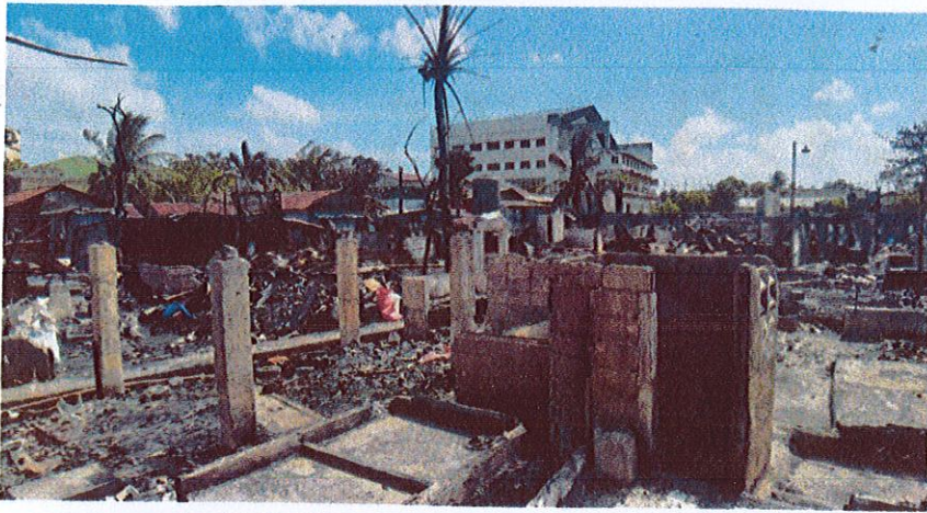
The day after the fire nothing was left
