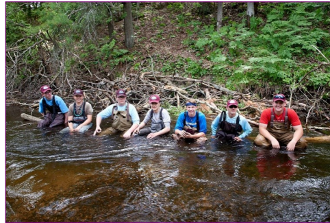
Improving trout habitat on the East Branch. A job well done.
