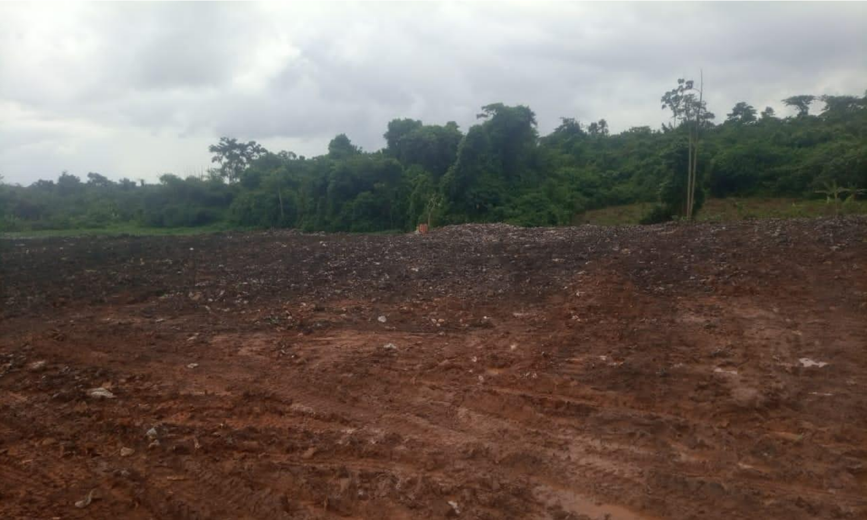
Final disposal site at Adankrono (After pushing and levelling)
