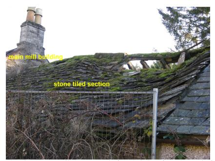
Plate 3. The stone-tiled (west) end of the building, from the north side, showing the partially collapsed roof. Water ingress and light conditions (both the ridge and the ceiling have large holes) make the area unsuitable for bat roosting.
