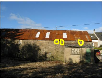
Plate 2. South face of the mill, showing a few deep holes in the stonework (circled) which are potential bat roosts, although no signs of roosts were found. Care should be exercised when repairing these holes.
