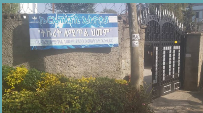
CareEpilepsy Ethiopia new office next to Denberwa MCH Hospital, Togo Street, Yeka Sub-City, Woreda 08, House No. 897, Addis Ababa
