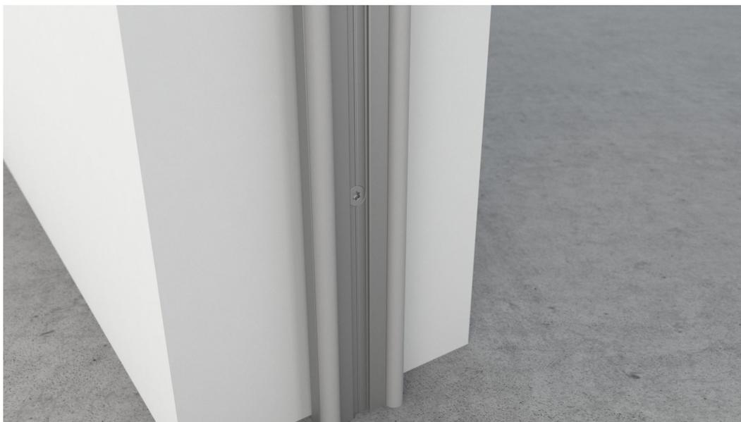
Fully tighten all screws, adjustments can be made when the door is installed.
