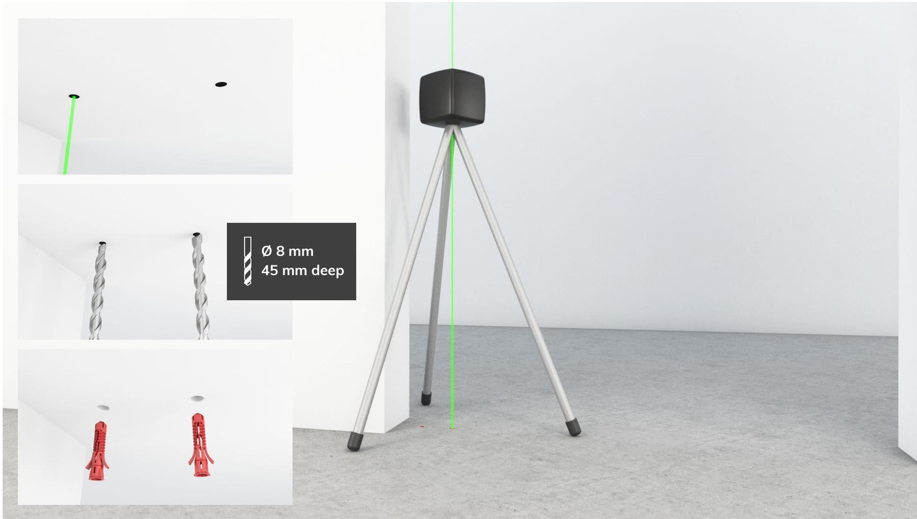
Use a laser to project and mark both holes to the ceiling. Drill holes and insert Hilti plugs.
