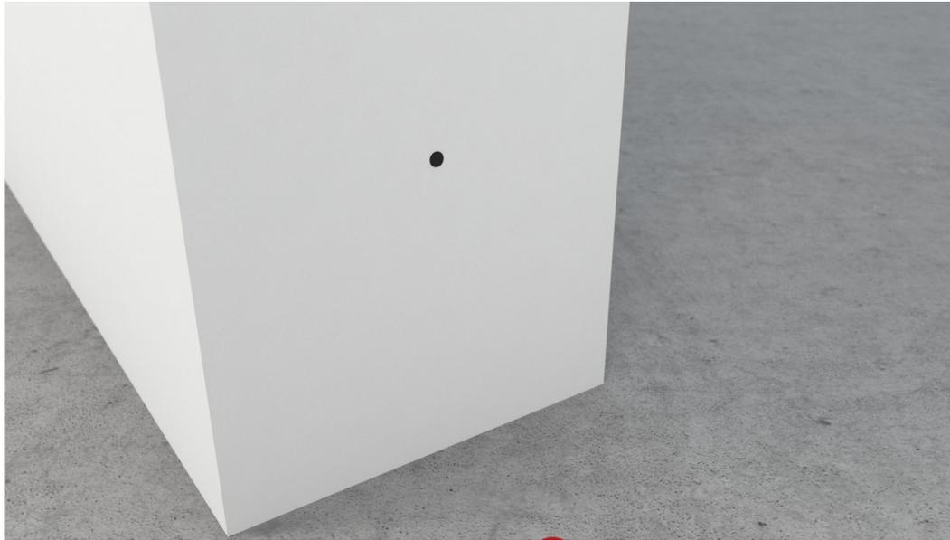
Drill all the holes in the marked locations, with a 6 mm drill +/-45 mm deep.
