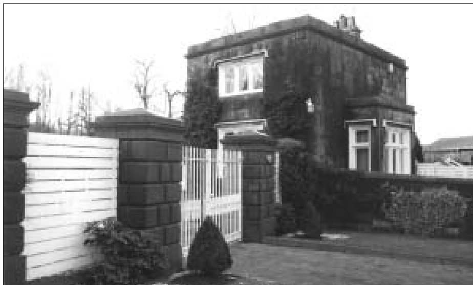
Winstanley Hall Lodge, Pemberton Road
