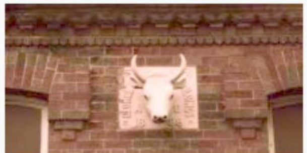
George Hampson's building 1888 ~ note the brick window hoods, typical of his properties.
