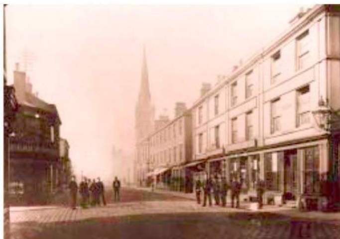
King Street with former Methodist Chapel spire. Note the former extent of the rendered terrace to the right partly replaced by the bank at Railway Road when it was widened.
