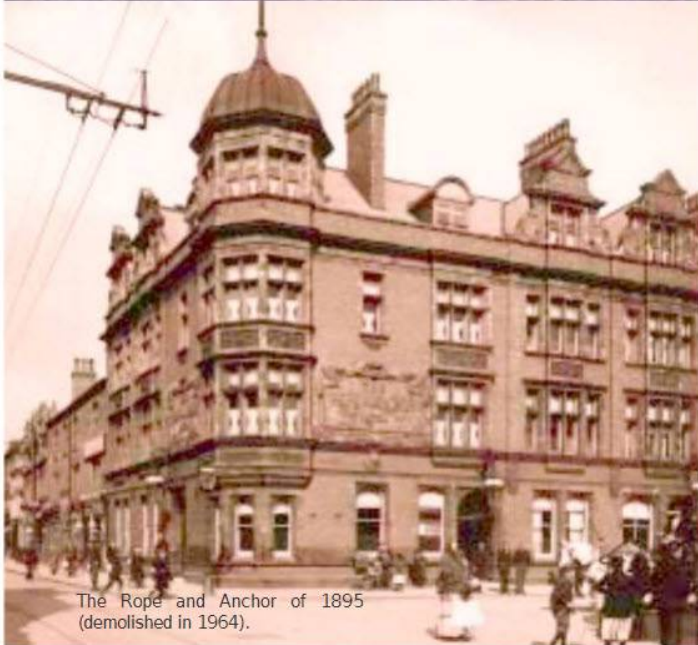
After 1863 the Rope and Anchor was extended to the corner until rebuilt in 1895.
