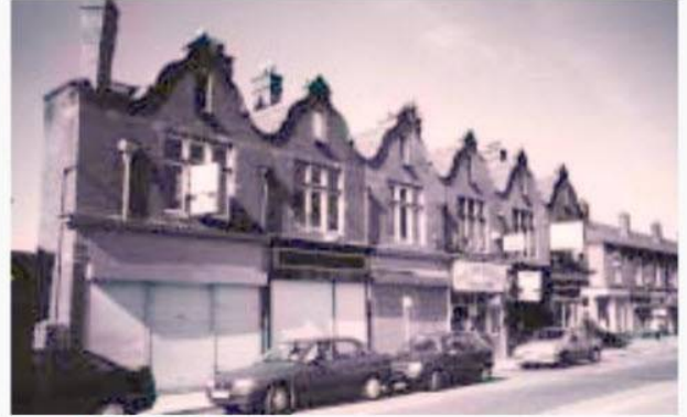
Railway Road shops with Dutch gables.
