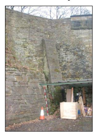
Figure 68 East-facing elevation of bridge over line of former rail route to foundry. Note multiphase construction- this section thought to have been re-built to accommodate trains
