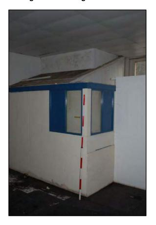
Figure 47 Building E: first floor window replaced with glass blocks, and internal wall surface plastered
