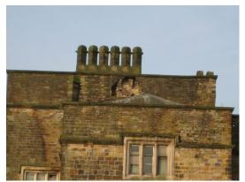
Void to masonry above tower back
