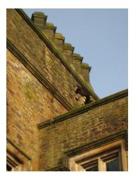
Dangerous loose masonry to tower
