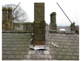
Roof from attic window: chimneys fixed to rotten timbers with steel ties.
