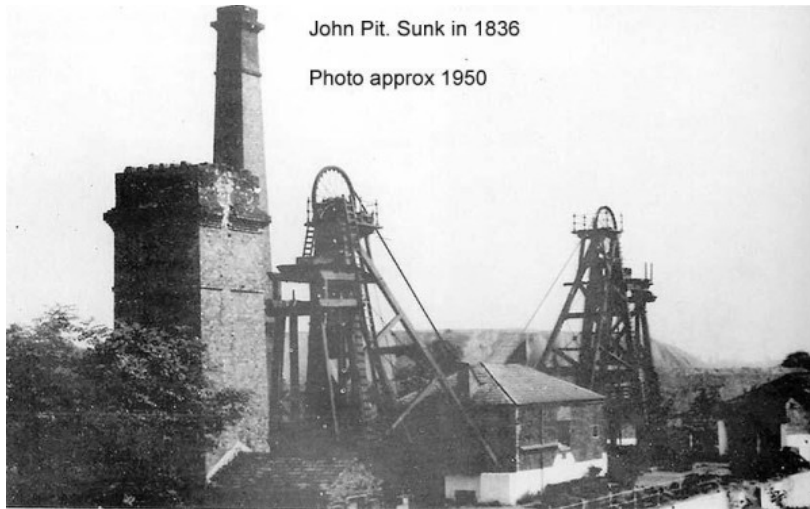
The John Pit, pit head and winding houses
