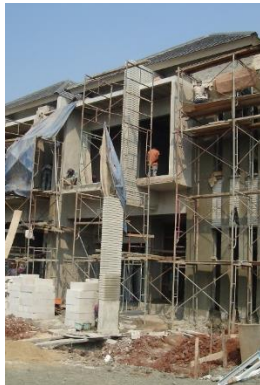
AAC Load Bearing Wall Grand Orchard Kelapa Gading Client: PT. Summarecon
