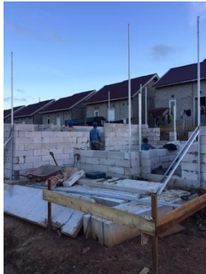
AAC Load Bearing Wall Batakan, Balikpapan
