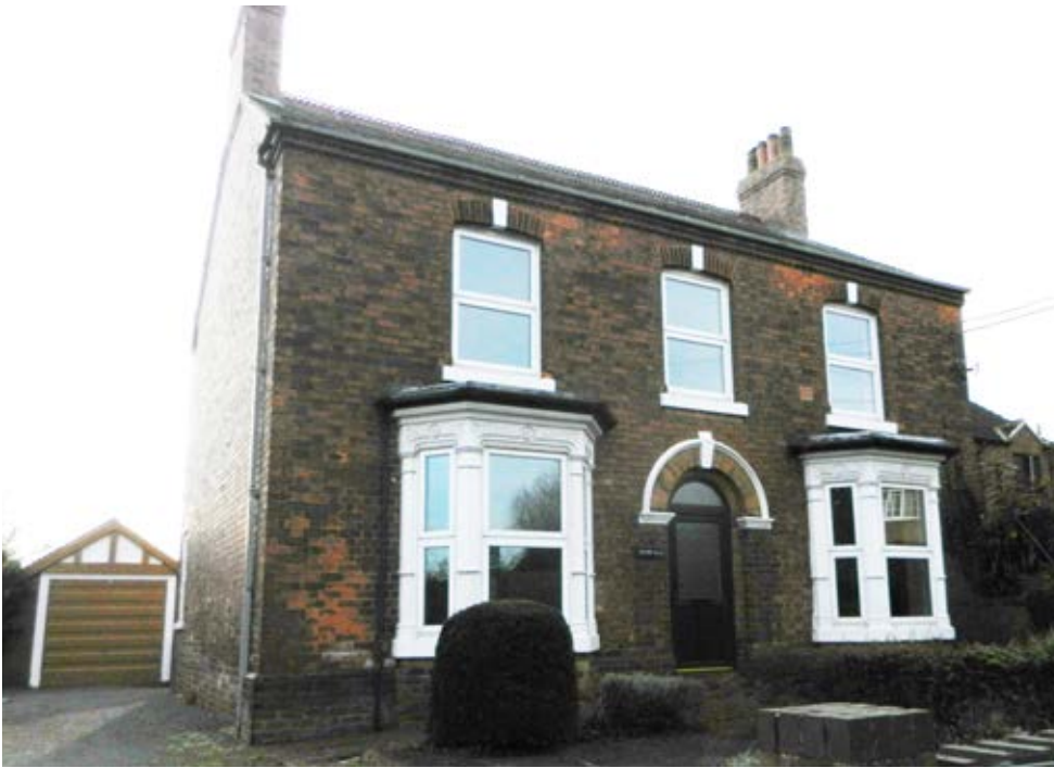
Figure 33: Bay windows and archway
