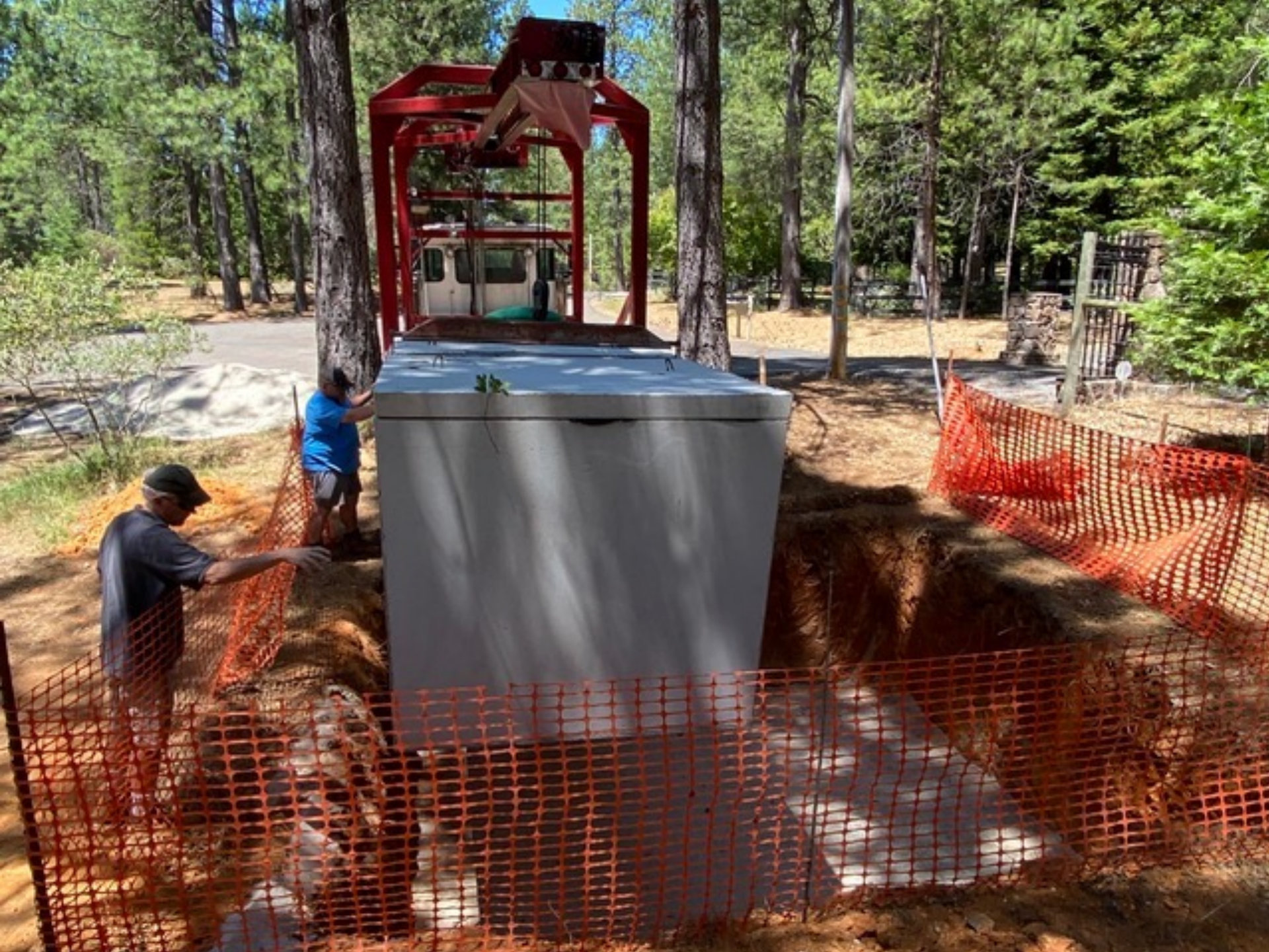
Concrete 2500-gallon tanks from Georgetown Precast
