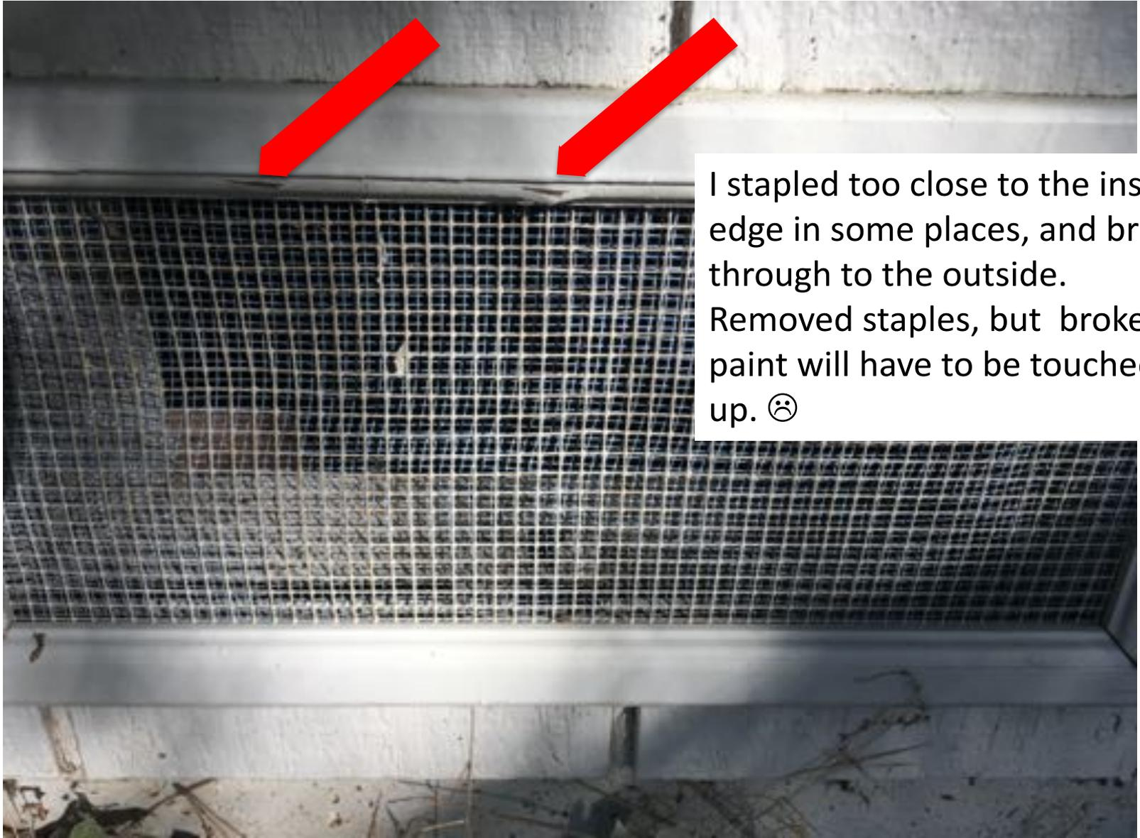
I stapled too close to the inside edge in some places, and broke through to the outside. Removed staples, but broken paint will have to be touched up. ☹️
