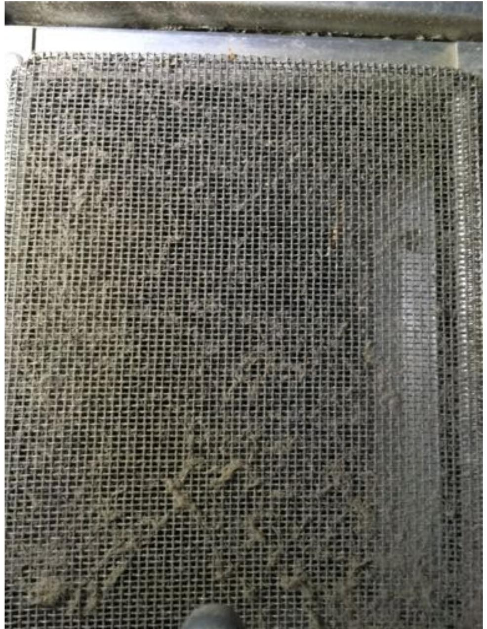
For gable vents, I cut 24" x 24" oversize mats for handyman to staple from the inside. I put blue masking tape on sharp raw wire edges to made them safer to handle in a difficult work environment.
