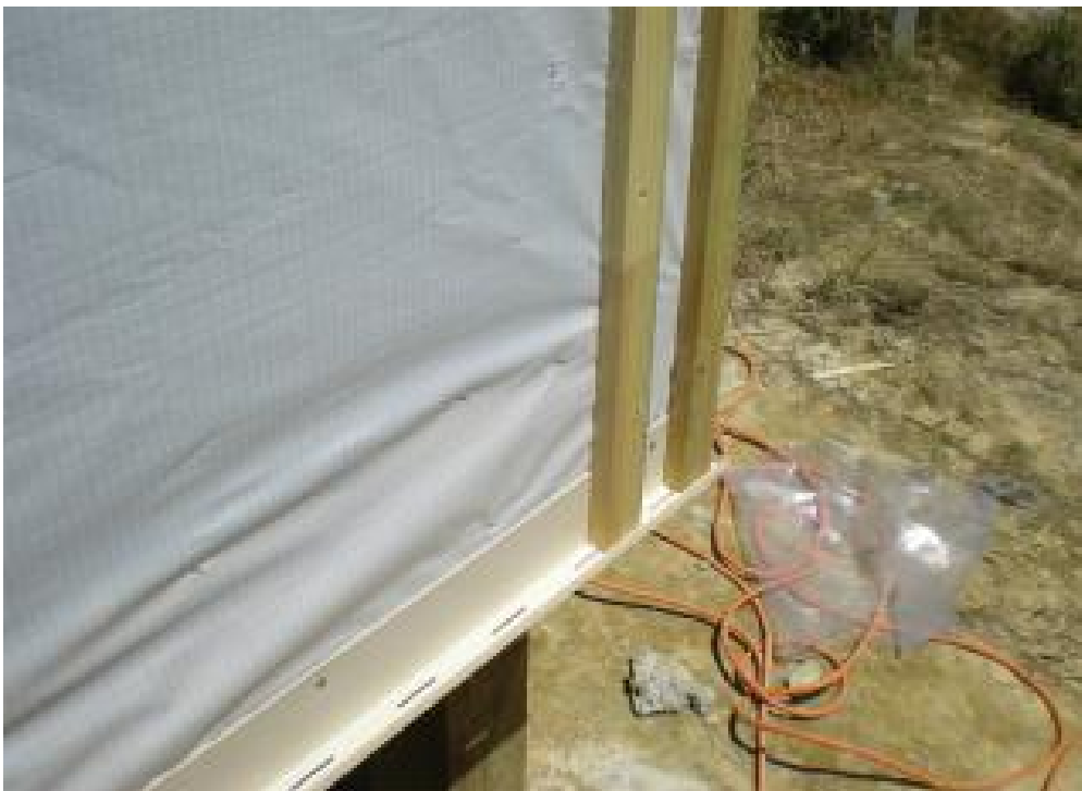
Drainage provided at the base of a wall cavity.
