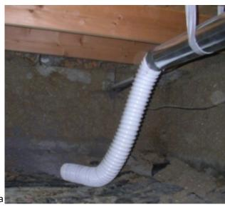
defective installation. They must terminate at the exterior and away from a door or window. Also, screens may be present at the duct termination and can accumulate lint and should be noted as improper.
