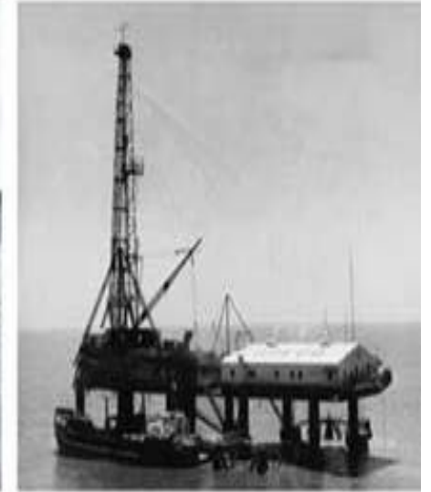
1953 - 'Mr. Charlie' offshore semisubmersible drilling unit and accommodation platform
